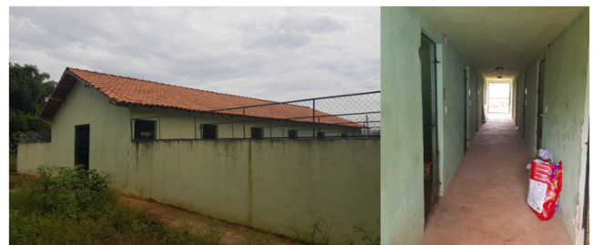
Fig. 1. Study building, its central corridor, and kennel doors.
